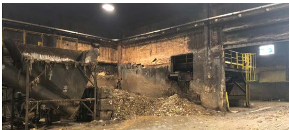
The truck loading station at the beginning of the project
