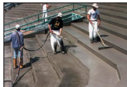
Concrete resurfacing.
