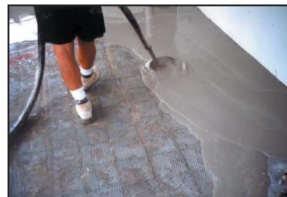
Self-leveling underlayments.
