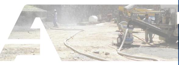
The Airplaco C-10HHD gunite machine provides maximum performance and efficiency due to its heavy-duty design and powerful output. The C-10HHD dry-mix shotcrete machine is exclusive to the gunite and shotcrete industry, offering a hydraulic motor to rotate the machine's feed system. C-10HHD gunite machines are typically used with batch plants, which provide a power-take-off (PTO) to motor on the shotcrete machine. The hydraulic motor reduces the overall amount
