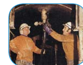
Grout injection and backfilling
